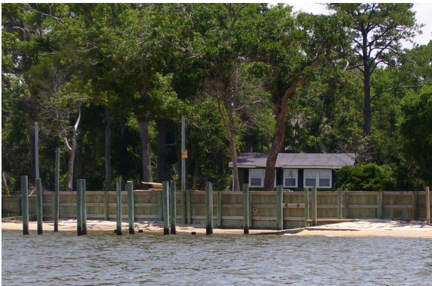
Figure 3.6 Groin and Bulkhead System by Mouth of Weeks Bay (~4km North of Study Area)
