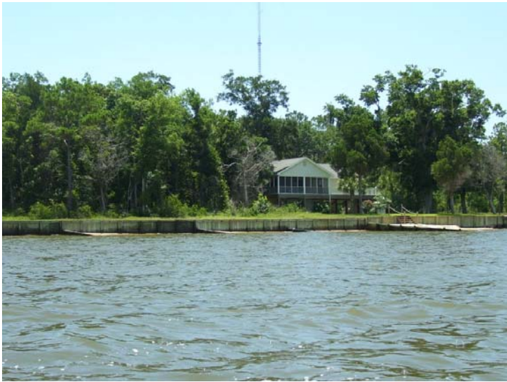
Figure 3.4 Bulkhead and Groin System ~3.5 km North of Study Area
