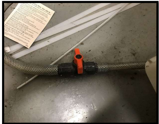
Figure 6: Salt water reservoir drainage valve (in the closed position as shown)
