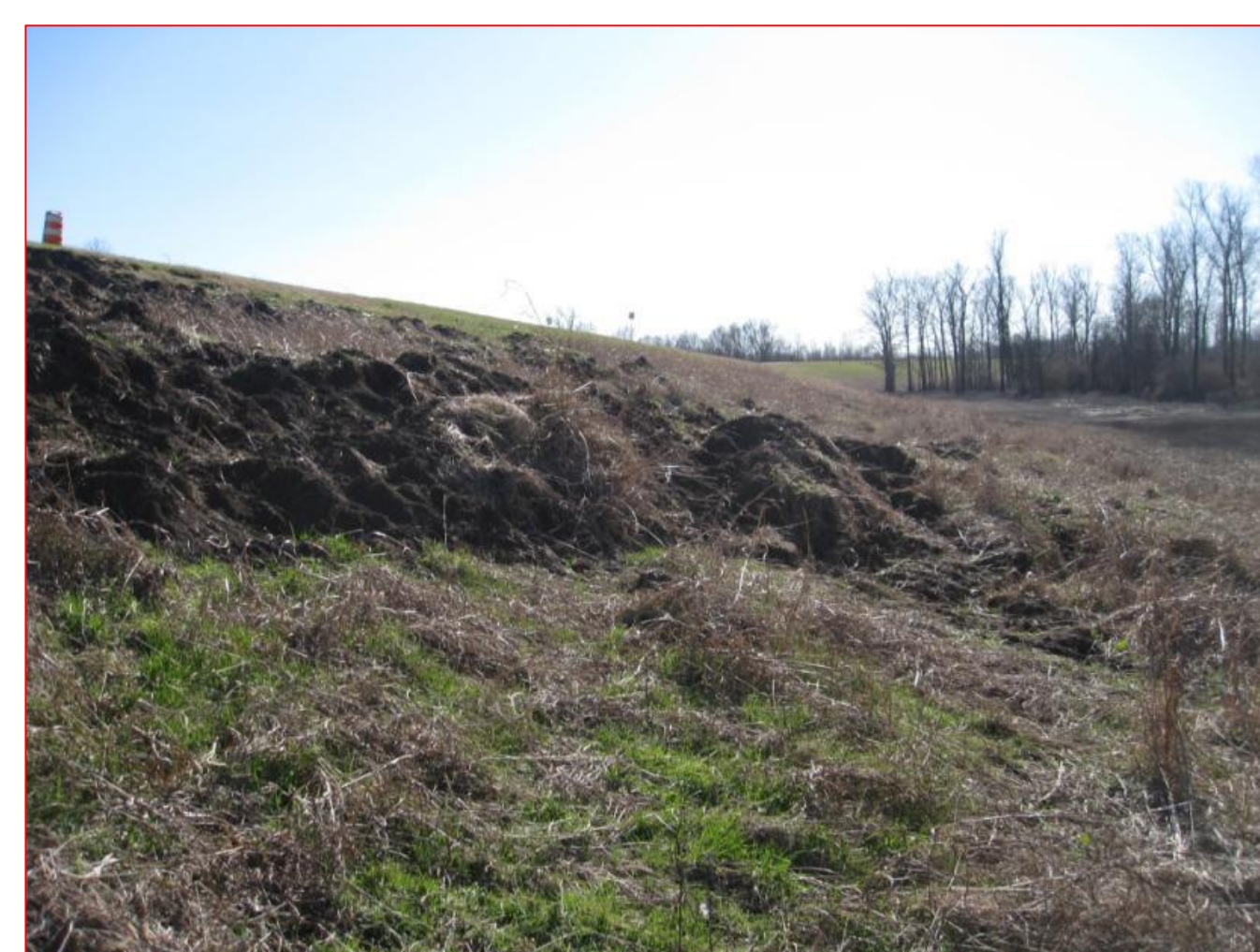
Fig 2: A Slump slide on the levee adjacent to Chotard Lake, MS, USA.
