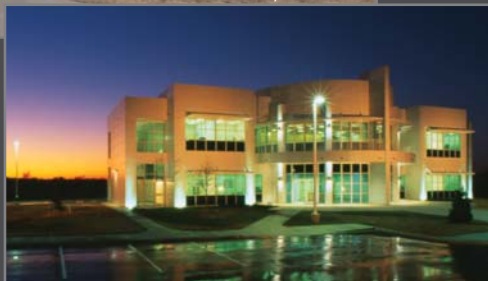
CAVS Extension Center in Canton
